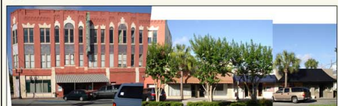
2 NEWCASTLE STREET (LOOKING EAST)
