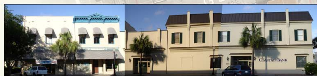
3 NEWCASTLE STREET (LOOKING EAST)
