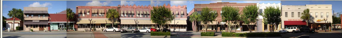
1 NEWCASTLE STREET (LOOKING EAST)
