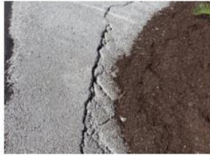
7 CRACKING-STRUCTURAL
