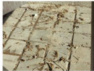
15 SEDIMENT (POOR)
