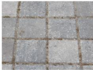
15 SEDIMENT (POOR)
