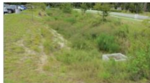
8 PRETREATMENT EROSION (SLIDE SLOPES) & 22 UNDESIRABLE VEGETATION (POOR)
