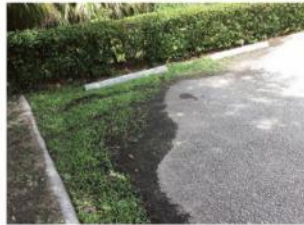
6 STANDING WATER, 12 VEGETATION (POOR) & 13 SEDIMENT (POOR)
