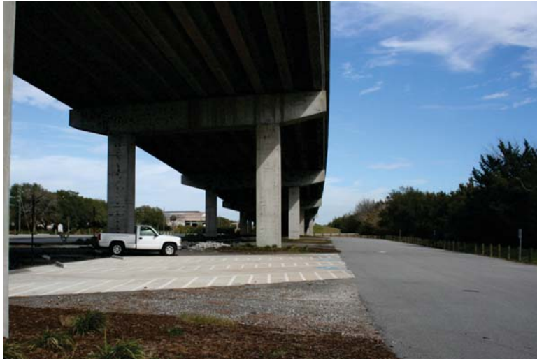
View looking North following overpass.
