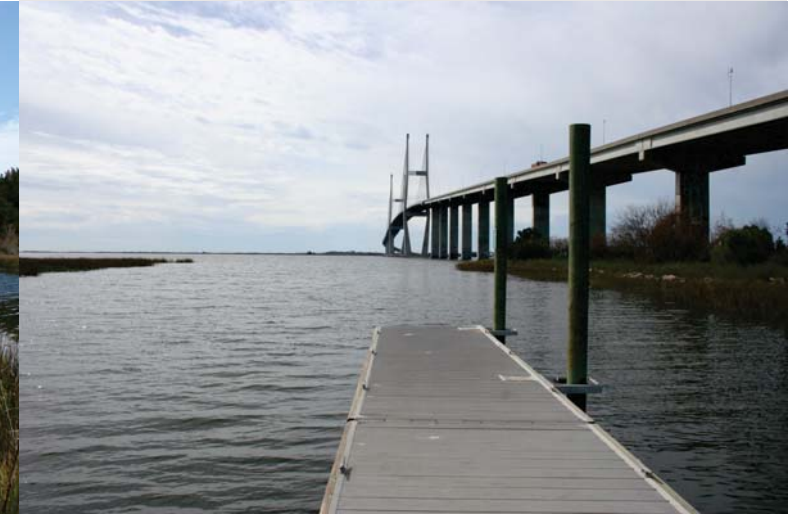
View from floating dock Sidney Lanier Bridge.
