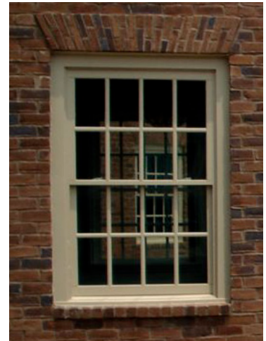
Brick Header and Sill
