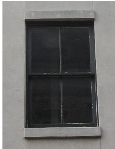
Stucco Header and Sill
