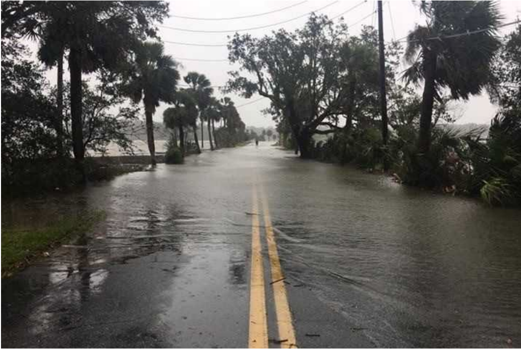
Figure 15: Burnside Island Causeway – Hurricane Irma (Photo Credit: Lindy Claborn / WJCL)
