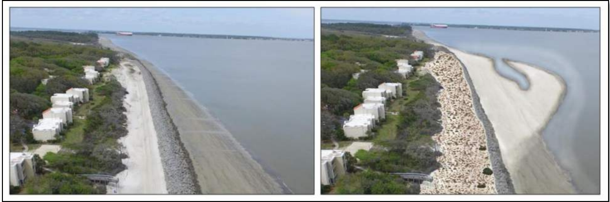
Figure 5.13: "Sand Motor" Project Visualization – Nearshore Placement
