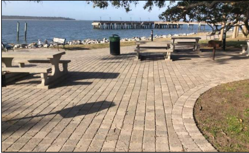
Figure 5.9: Permeable Pavement at Neptune Park, near St. Simons Island Fishing Pier.
