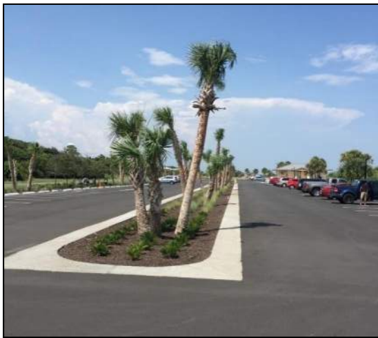
Figure 5.10: Oceanview Beach Park GI/LID Practices – Bioretention with Pervious Concrete Border (left) and Constructed Stormwater Wetland (right).
