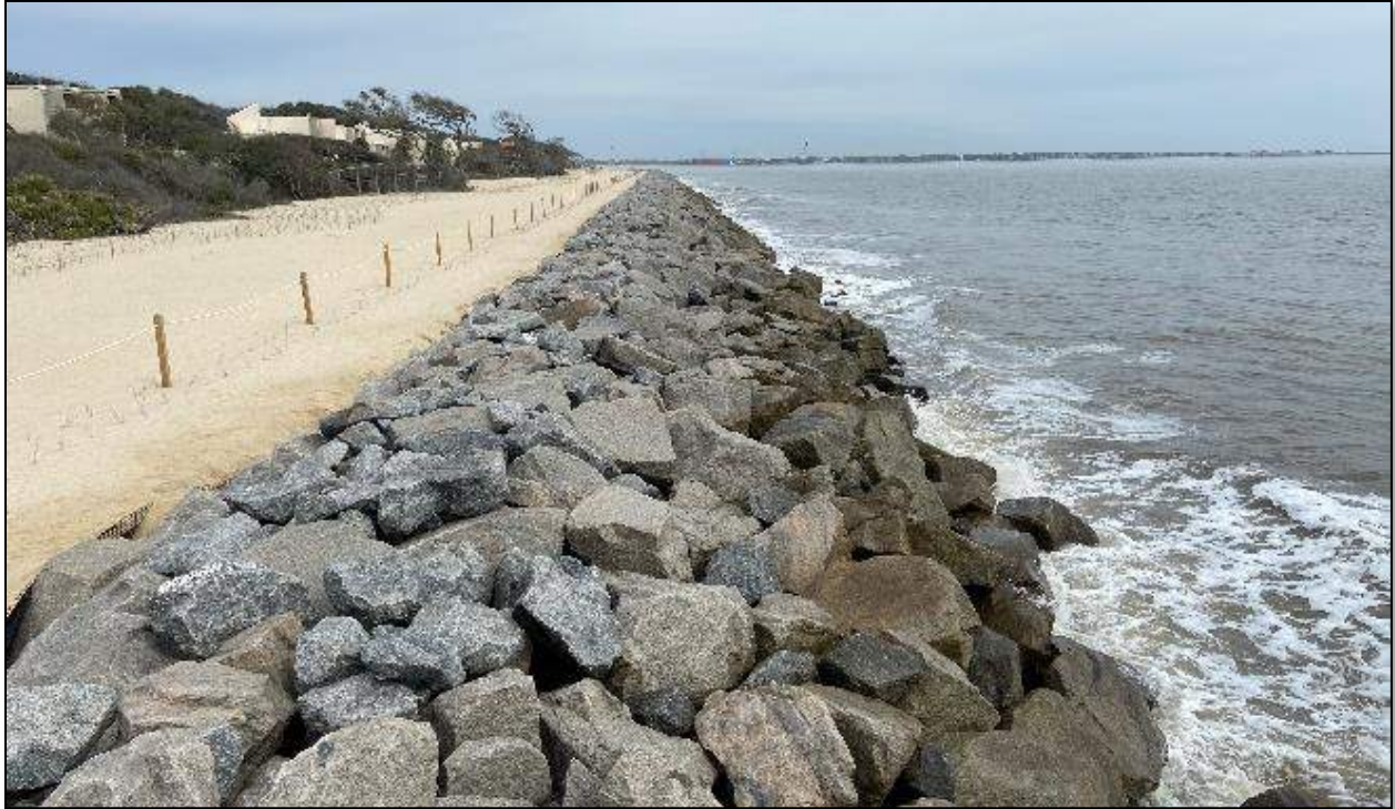
Figure 5.12: Recently Completed Rock Revetment Project on Jekyll Island.
