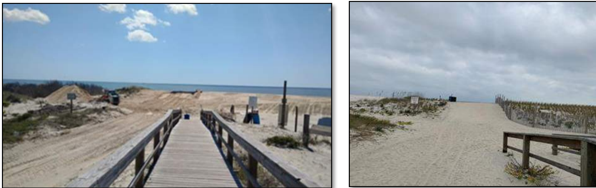
Figure 2.4: Before (left) and After (right) of PermaShield™ Constructed Dune on Tybee Island. Photo Credit: Guardian Retention Systems
