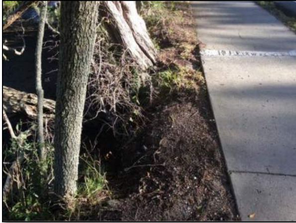
ID: #GI-14 – St. Simons Island, Ocean Blvd. Headwall Erosion
