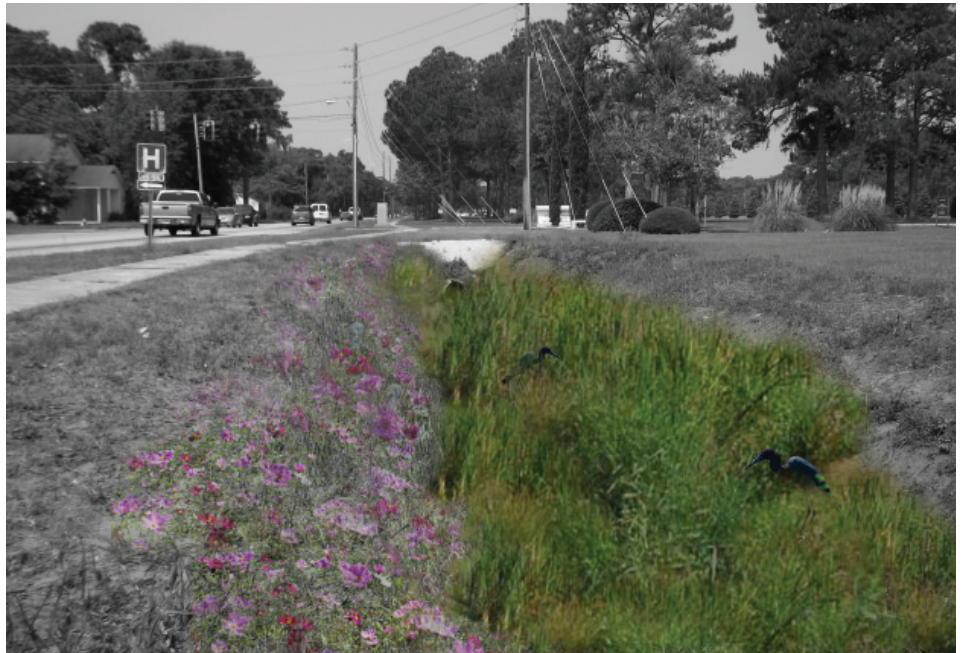
Improvements to the bioswale along Fourth Street
