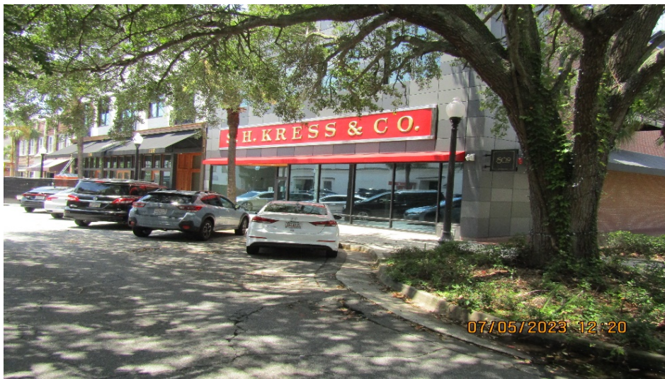
The recently completed repurposed Kress Hotel in Downtown Brunswick
