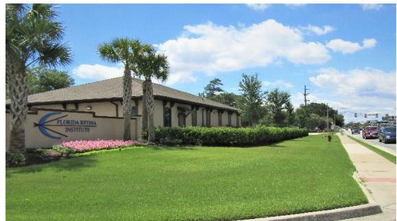
New construction - medical services building on Glynn Avenue
