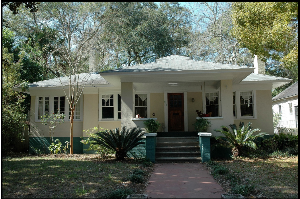
Photo 20: Prairie style bungalow – 917 Egmont Street (1915-19)
