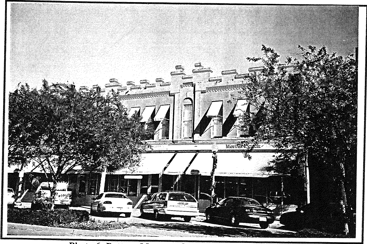
Photo 6: Pattern Masonry Queen Anne, Hotel Royal, 1616 Newcastle Street (c1899-1907) – GN-B-11
