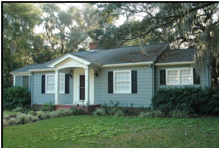
Photo 18: 20126 Ash Ave. (c1939-40) – Windsor Park
