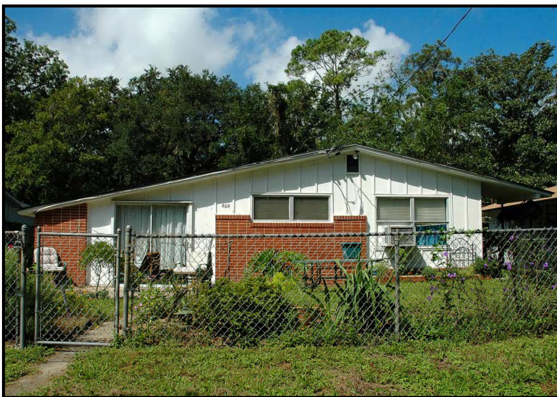
Photo 2: 809 Gordon Street (c1955-64) – Habersham Park
