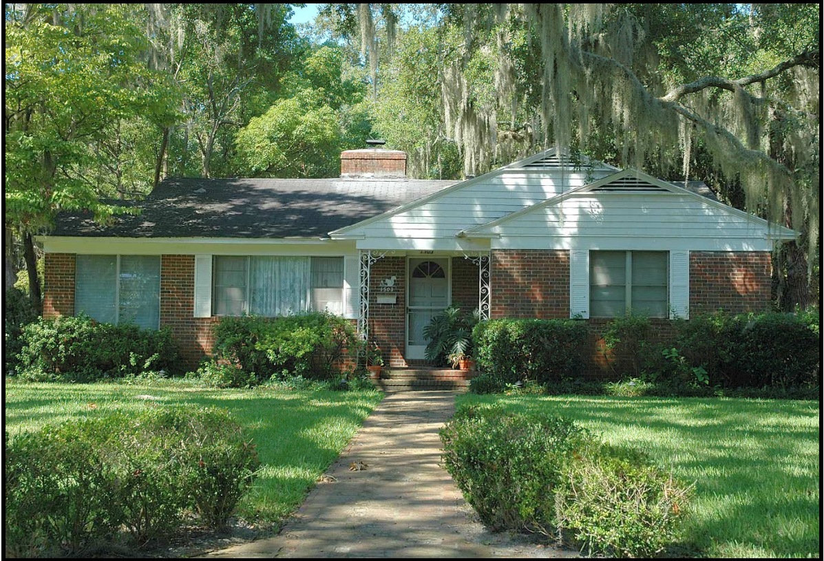
Photo 46: 1303 Sycamore Avenue (c1949) – Windsor Park Subdivision
