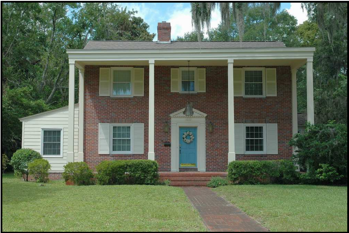
Photo 33: 1227 Sycamore Avenue (c1937-38) – Windsor Park Subdivision
