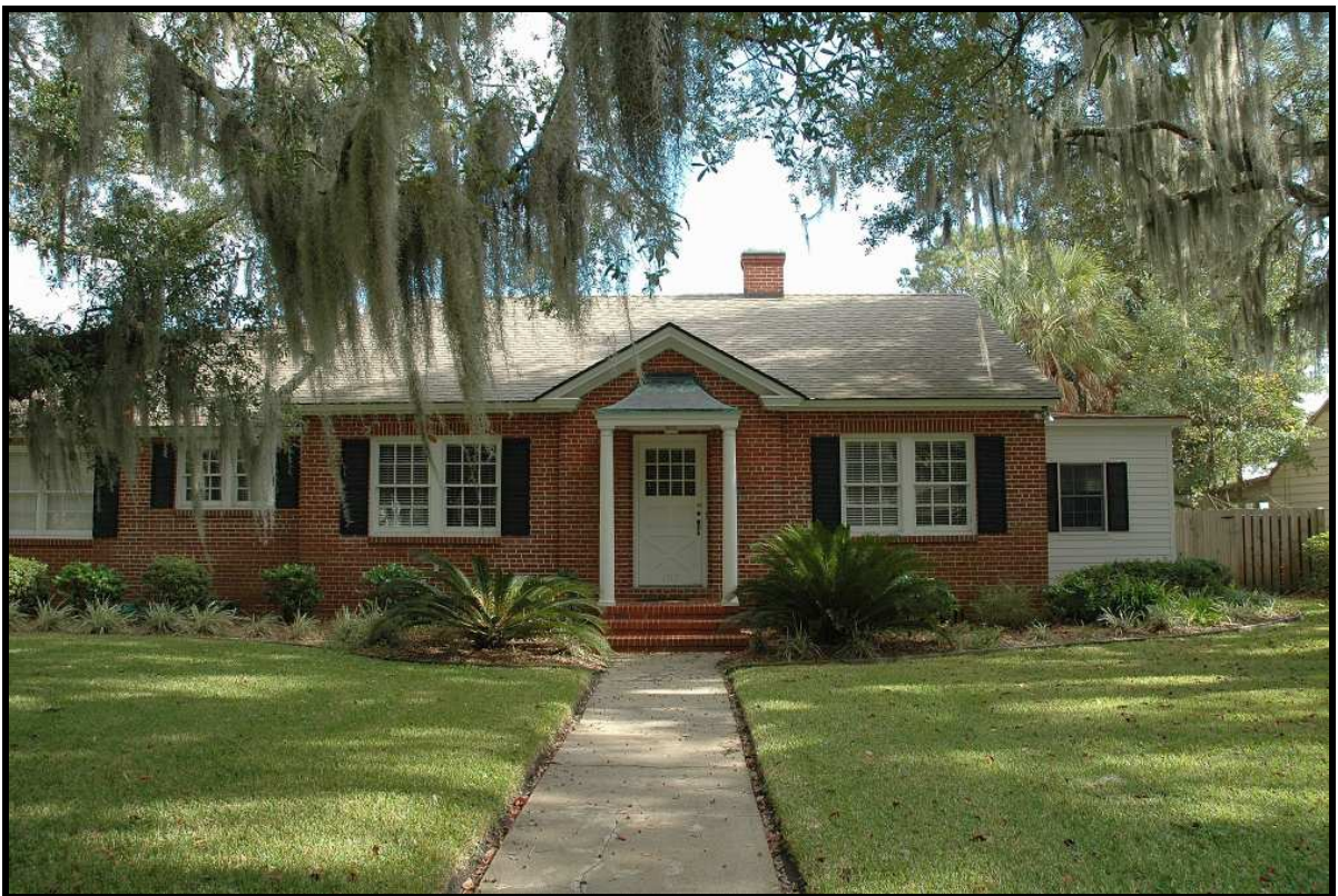
Photo 44: 1312 Palmetto Avenue (c1941-43) – Windsor Park Subdivision
