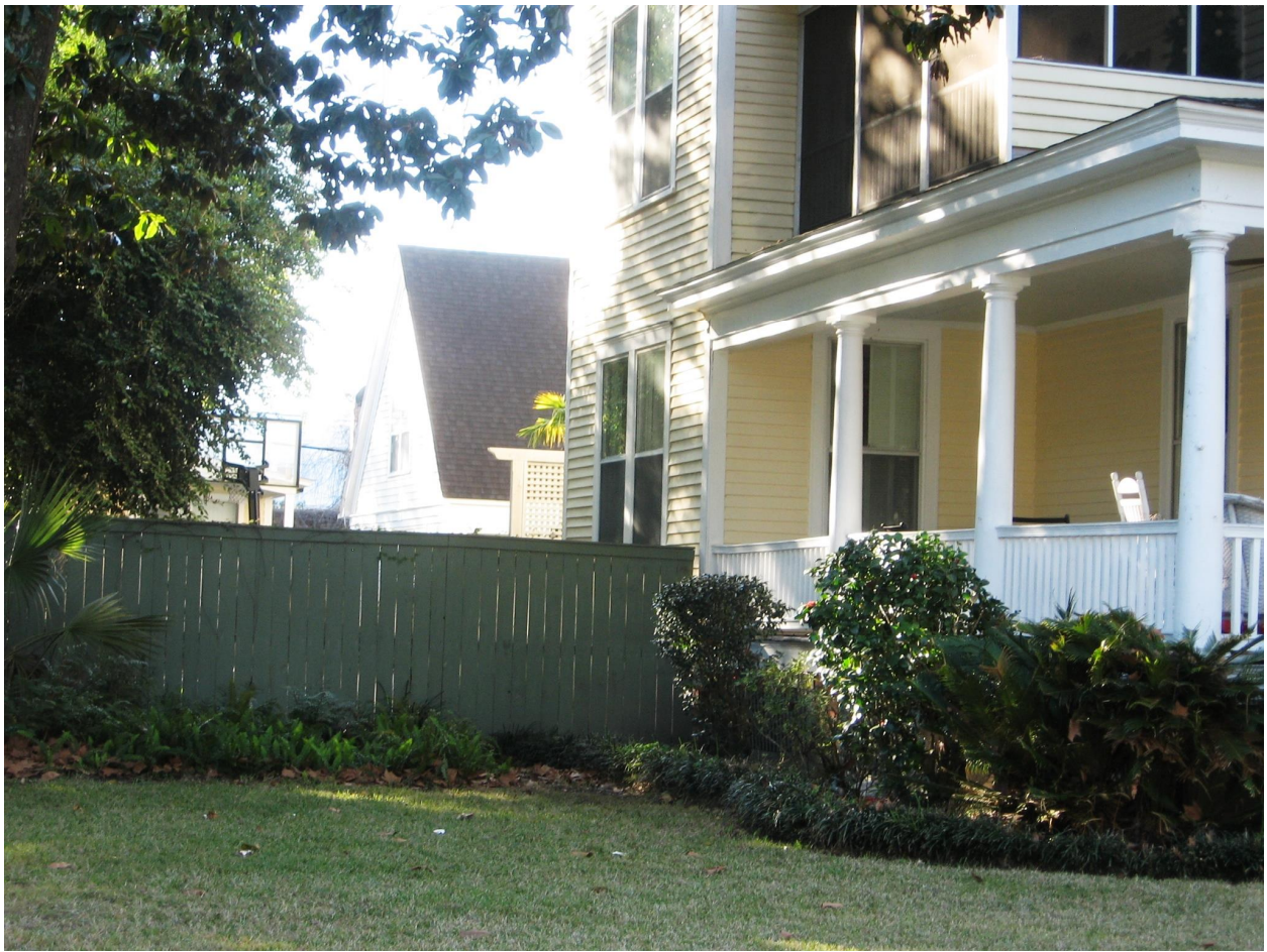
The privacy fence at 1027 Union Street is appropriately recessed from the front of the house and has compatible height and materials.
