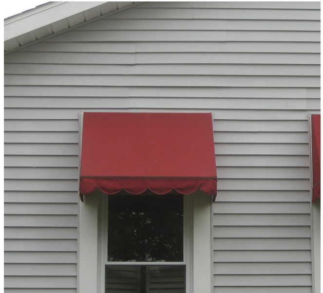
These examples of appropriate window awnings are of canvas material and of shed design. The awning pictured above left is designed to cover paired connecting windows while the other is correctly sized to the window opening.
