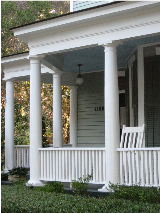
By the early 1900s many dwellings were built with classical columns such as the Tuscan porch columns at 1120 Union Street (left) and the Corinthian columns at 825 Egmont Street (right).
