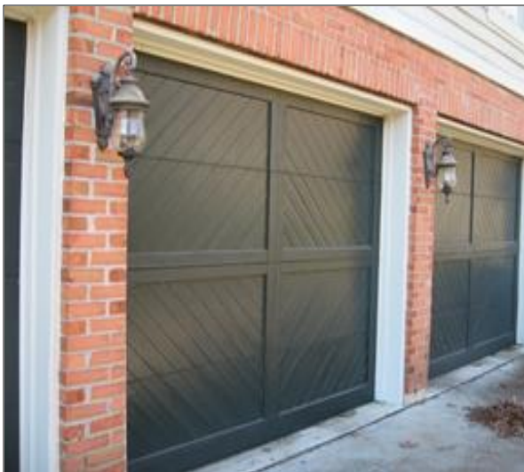
If replacement garage doors are needed on garages, sectional roll-up doors in traditional designs are appropriate.
