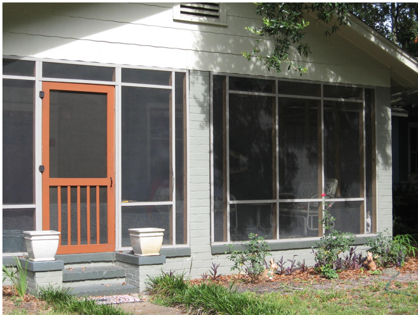
This porch at 805 Albany Street illustrates an appropriate amount of structural framework for screening in porches.
