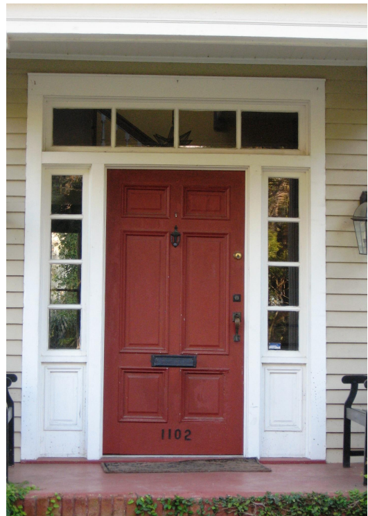
Original six-panel wood door with a multi-light transom and sidelights (1102 Prince Street).
