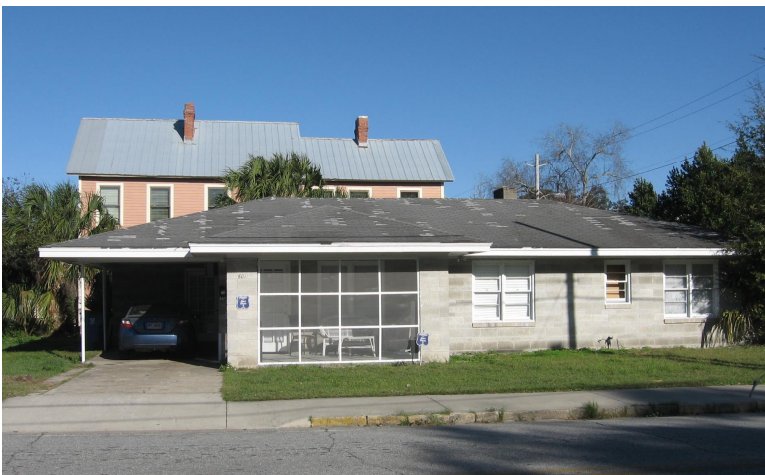
The exterior of this Ranch style dwelling at 601 F Street has an exterior of unfinished concrete that should be maintained and preserved in its original condition and not painted.
