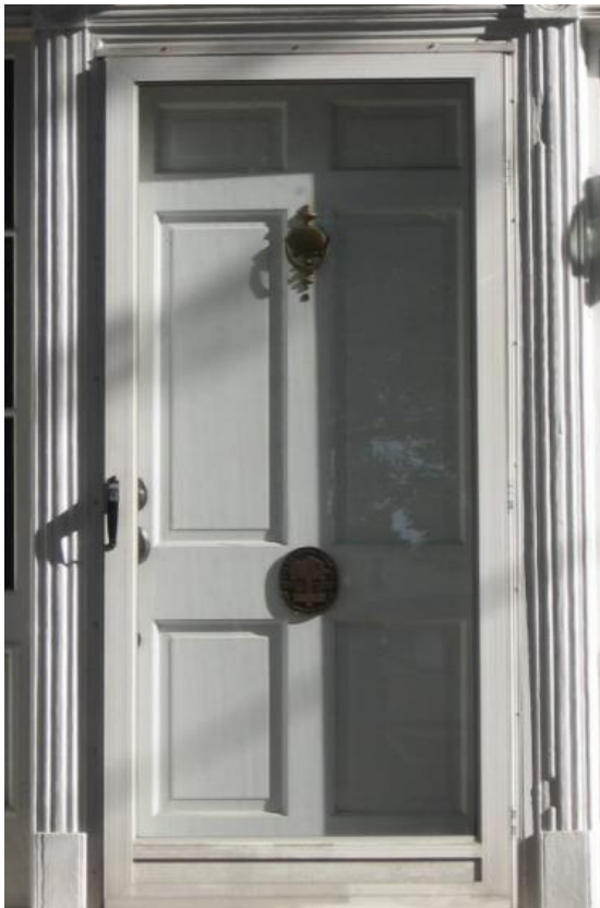
Storm doors may be added to primary entrances if they are full-view design.
