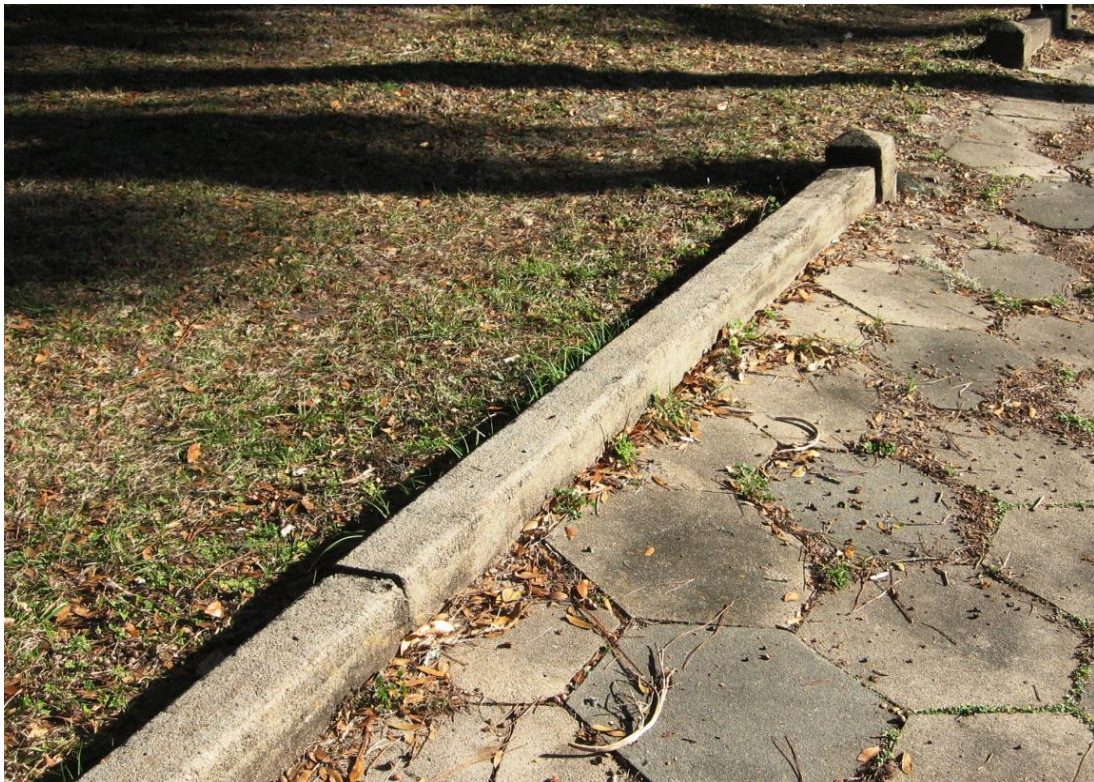
Several dwellings display early 20th century concrete retaining walls (above, 1027 Union Street) and walkway curbing (below, 528 Union Street). These features should be retained and not altered or removed.
