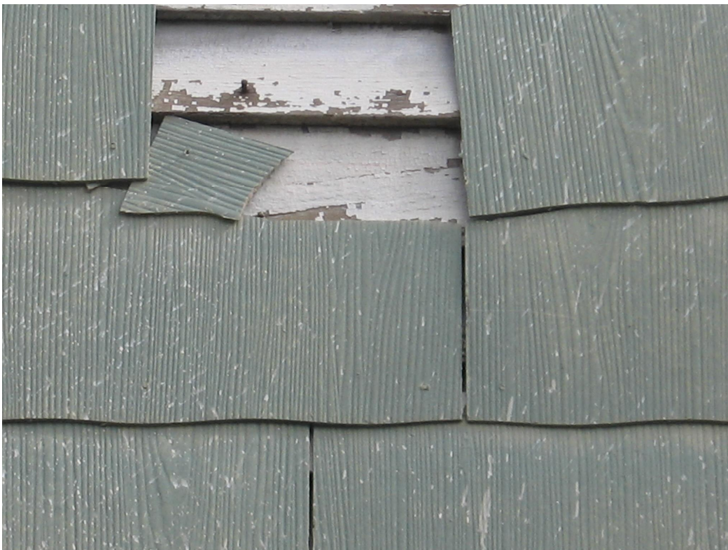
Several dwellings in the historic district have asbestos shingles added over the original wood siding. Removal of the shingles and restoration of the siding is encouraged (above 602 Dartmouth Street and below 1315 Union Street).
