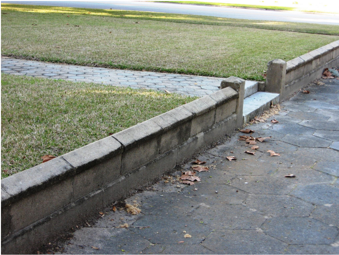
Several dwellings display early 20th century concrete retaining walls (above, 1027 Union Street) and walkway curbing (below, 528 Union Street). These features should be retained and not altered or removed.
