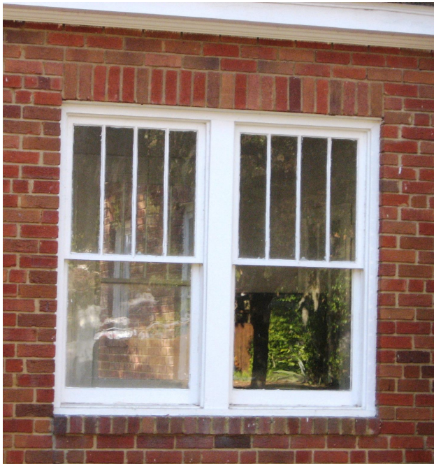
Craftsman style dwellings often features vertical lights in the upper sash as at 607 Union Street.
