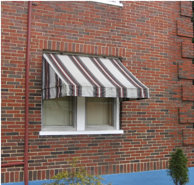
These examples of appropriate window awnings are of canvas material and of shed design. The awning pictured above left is designed to cover paired connecting windows while the other is correctly sized to the window opening.
