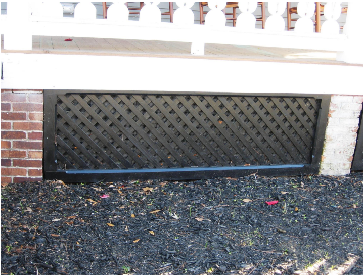
The placement of lattice panels between brick piers is appropriate if they are traditional design and recessed from the face of the pier (928 Union Street).
