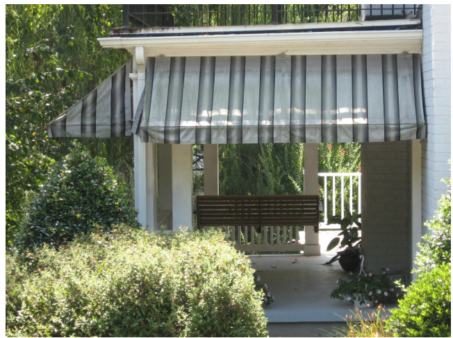
These examples of appropriate porch awnings are of shed design and of canvas material. They fit the porch opening and do not conceal architectural details.
