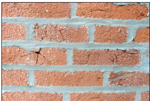
Abrasive cleaning of brick removes the exterior “crust” and can lead to deterioration as shown at left and spalling as shown at right.
