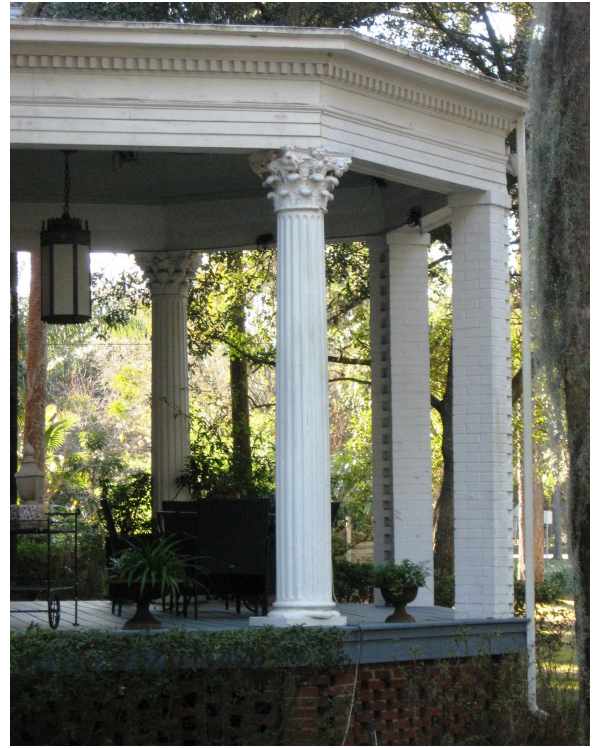
By the early 1900s many dwellings were built with classical columns such as the Tuscan porch columns at 1120 Union Street (left) and the Corinthian columns at 825 Egmont Street (right).
