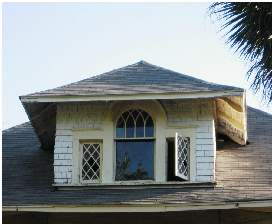
Windows may also be located in roof dormers and these are sometimes decorative in design. This dormer window is known as a Palladian design with its central arched sash and flanking rectangular casements.
