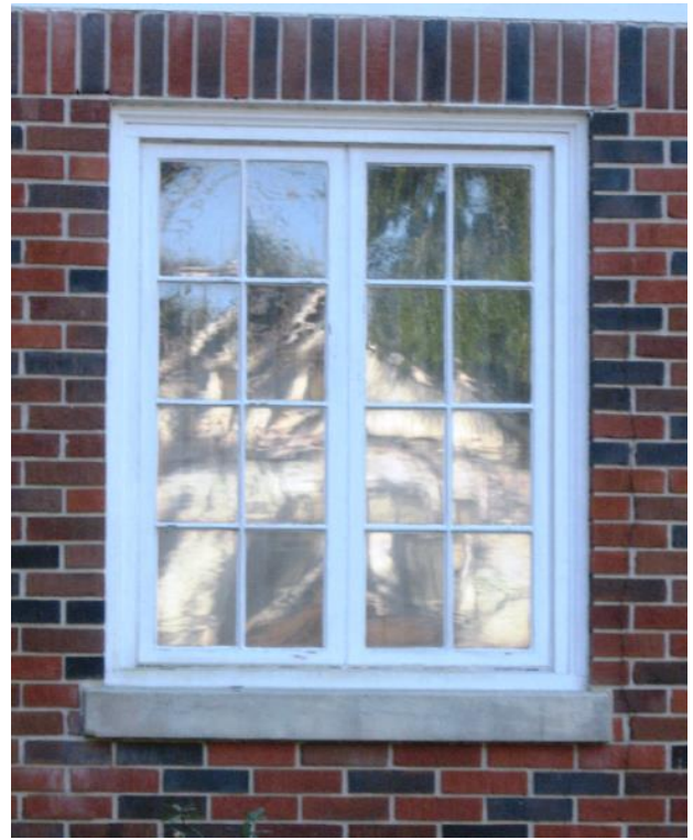
Preserve and maintain original window materials and designs. At left is an original two-over-two wood sash window at 927 927 Union Street. Dwellings may also display wood or metal casement windows as at 509 Union Street (right).
