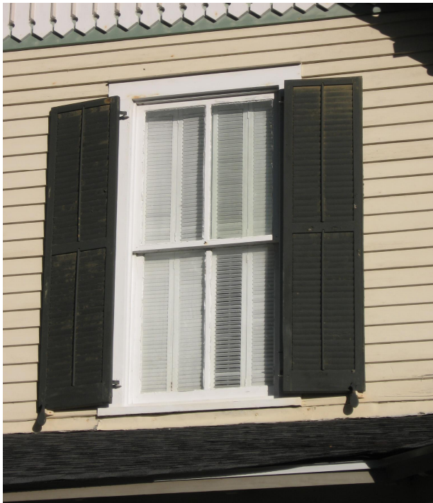
These original sash windows have appropriately designed and placed shutters which can be closed to protect the windows during storms (left, 903 Monck Street and right, 706 Union Street).
