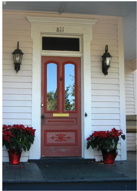
The entrance at 811 Union Street has an original two-arched-light door, transom, and surround.
