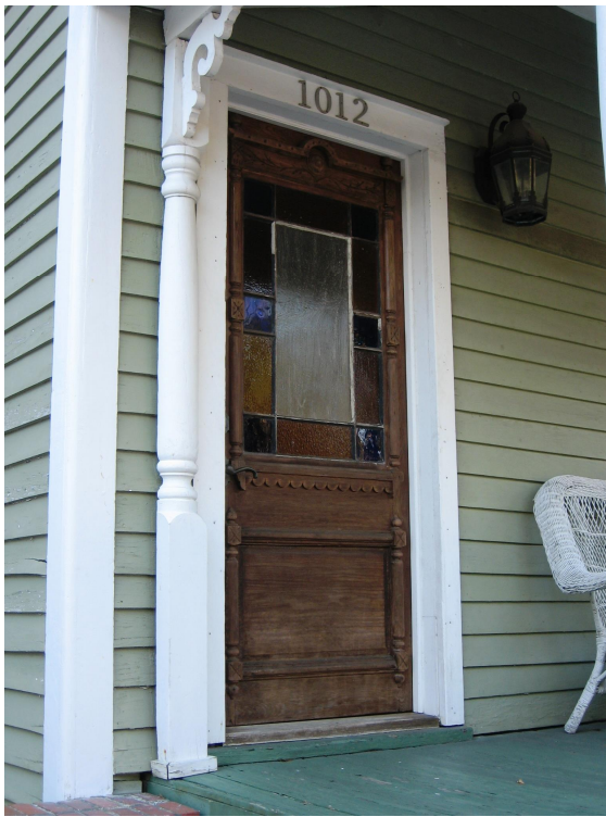
This entrance retains its original door with multi-colored border glass (1012 Carpenter Street).
