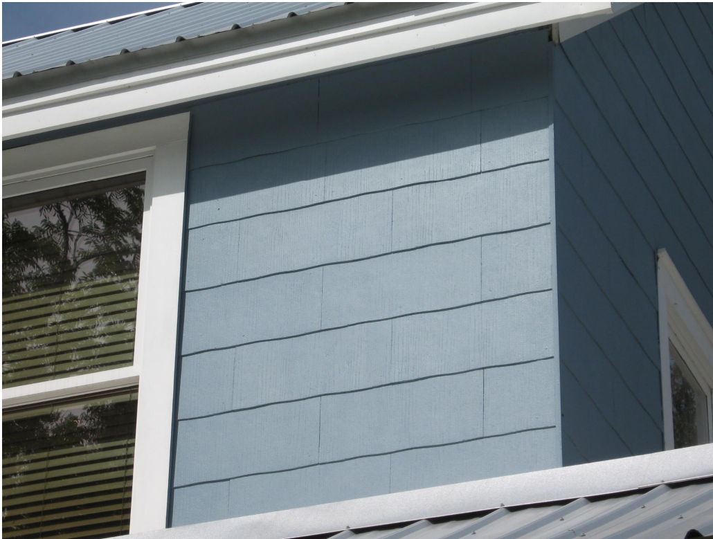
Several dwellings in the historic district have asbestos shingles added over the original wood siding. Removal of the shingles and restoration of the siding is encouraged (above 602 Dartmouth Street and below 1315 Union Street).
