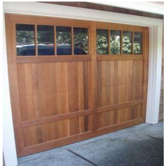
If replacement garage doors are needed on garages, sectional roll-up doors in traditional designs are appropriate.
