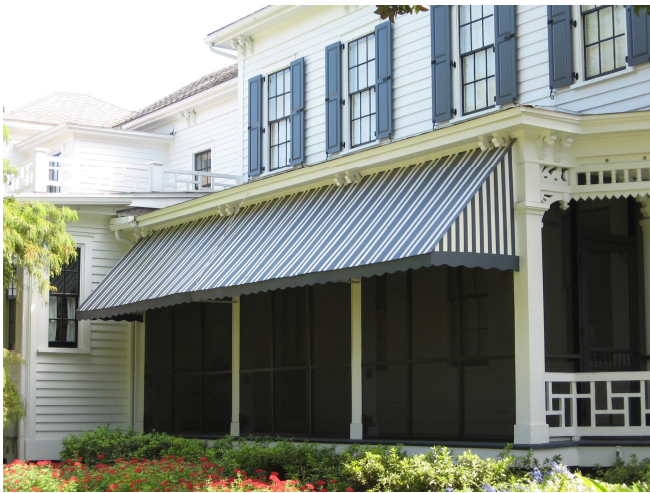
These examples of appropriate porch awnings are of shed design and of canvas material. They fit the porch opening and do not conceal architectural details.
