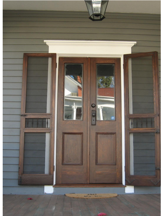
The entrance at 3 Halifax Square has original screen doors which reflect the historic door they cover.
