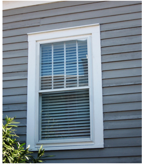
This full-view storm window assists in energy efficiency but allows viewing of the original window behind it (600 Mansfield Street).
