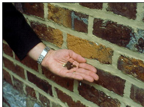
Abrasive cleaning of brick removes the exterior “crust” and can lead to deterioration as shown at left and spalling as shown at right.
