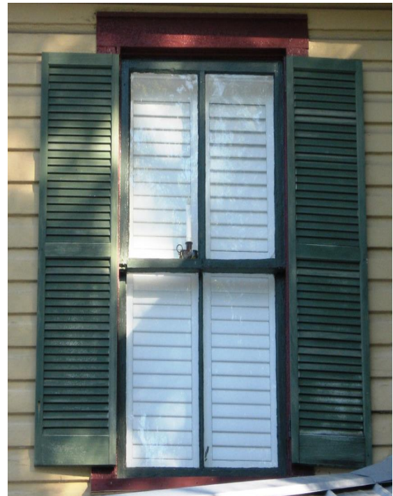
These original sash windows have appropriately designed and placed shutters which can be closed to protect the windows during storms (left, 903 Monck Street and right, 706 Union Street).
