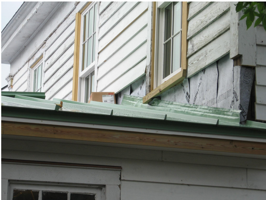
New metal standing seam roofs should have seams that are no more than 1" in profile as in this roof.
