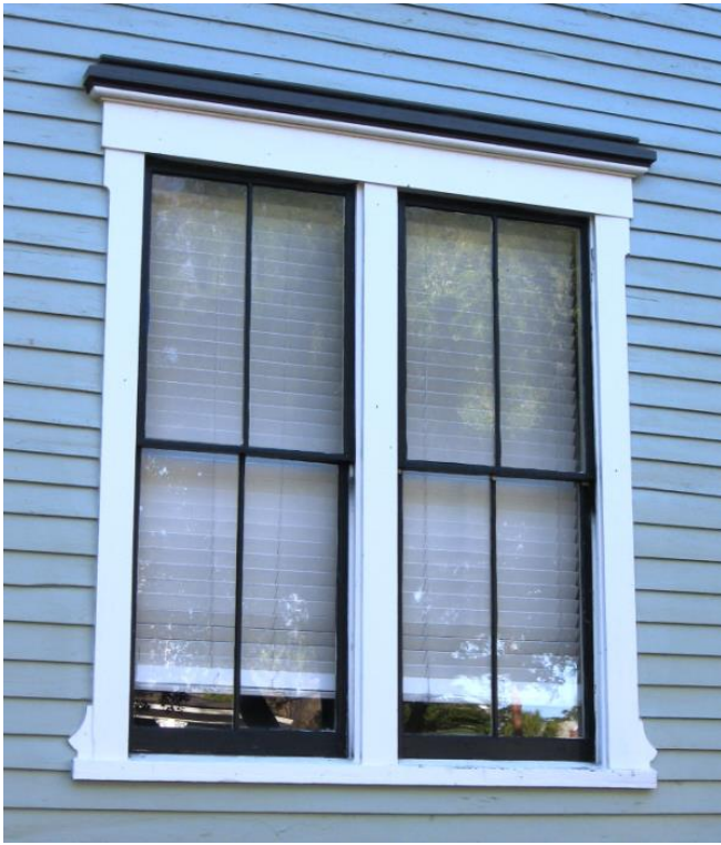
Preserve and maintain original window materials and designs. At left is an original two-over-two wood sash window at 927 927 Union Street. Dwellings may also display wood or metal casement windows as at 509 Union Street (right).
