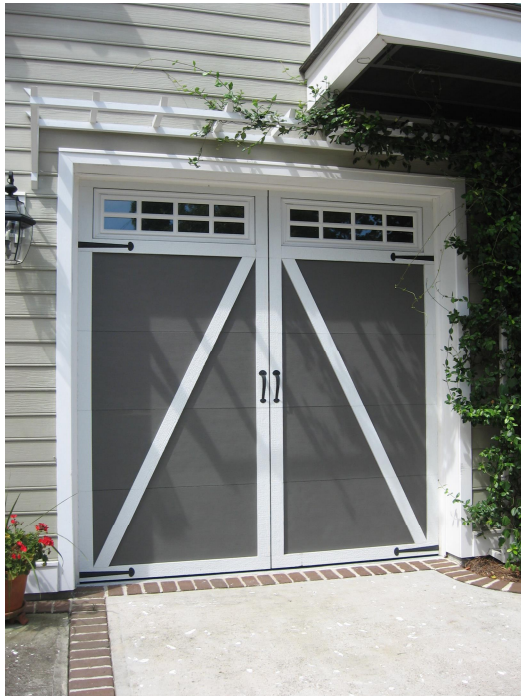
Garage doors should be in traditional designs such as paneled wood, glass and wood, and diagonal board such as on this new garage.
