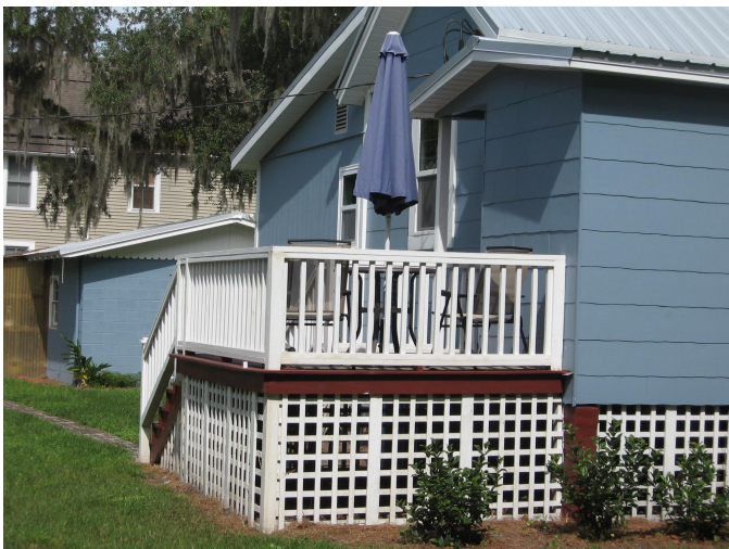
Example of an appropriately located and sized rear deck with square wood balusters at 602 Dartmouth Street.
