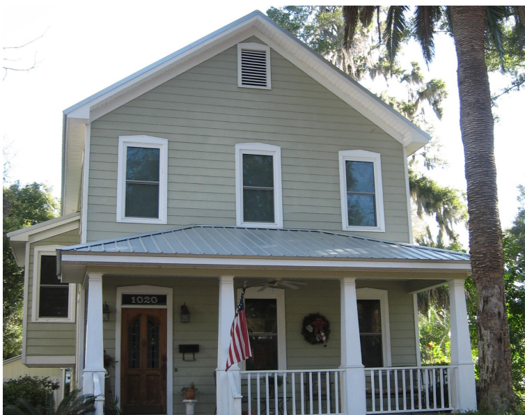
This infill dwelling constructed in 1993 at 1020 Union Street is an appropriate imitation of a historic house type with its gable-front form, façade arrangement, porch dimensions, and window configuration.
