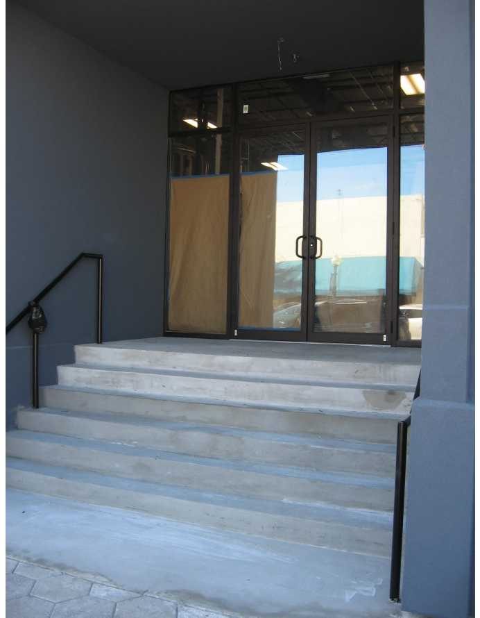
The new building at 1325 Newcastle Street was designed with elevated concrete bulkheads and a raised stair entrance to withstand flooding.
