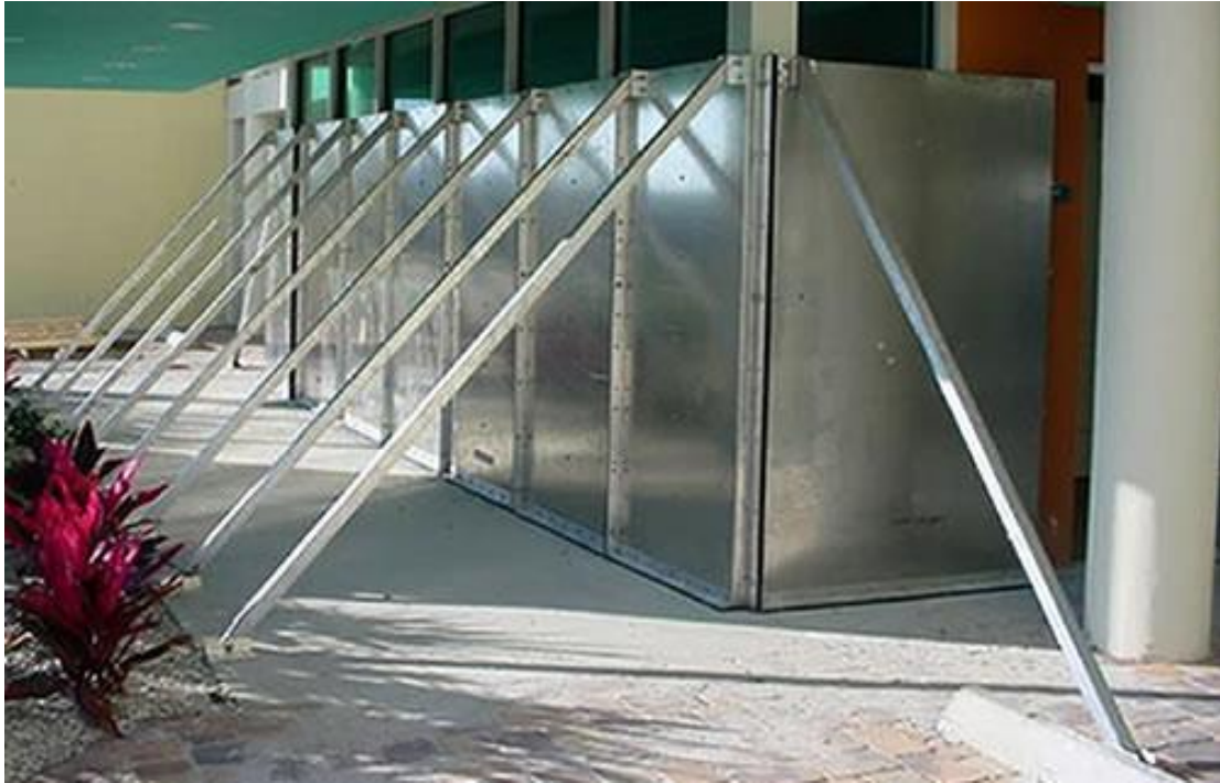
Temporary flood panels are now widely available for historic commercial buildings. When high water events are anticipated these can be erected to minimize flood damage.
