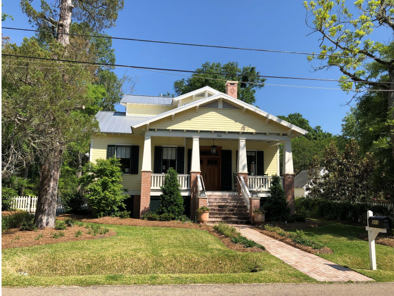
When elevating dwellings the porch columns may be extended on brick piers with lattice panels between the piers.
