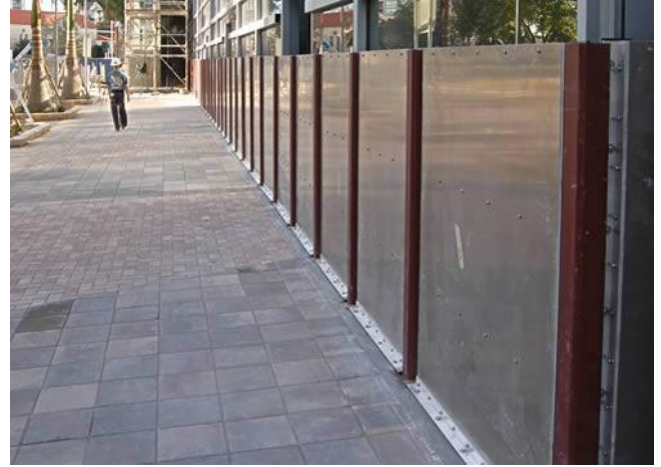
Temporary flood panels are now widely available for historic commercial buildings. When high water events are anticipated these can be erected to minimize flood damage.
