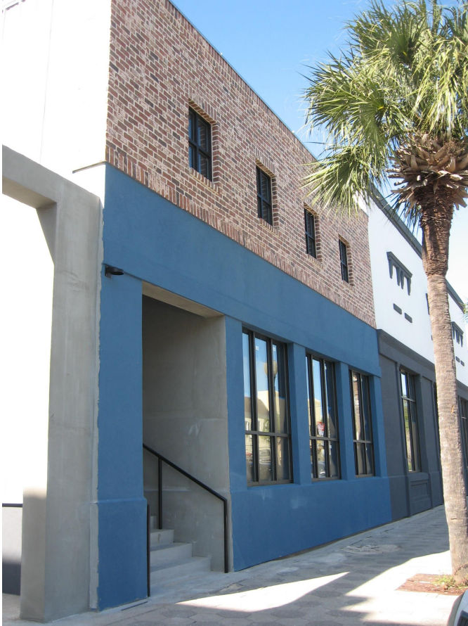
The new building at 1325 Newcastle Street was designed with elevated concrete bulkheads and a raised stair entrance to withstand flooding.
