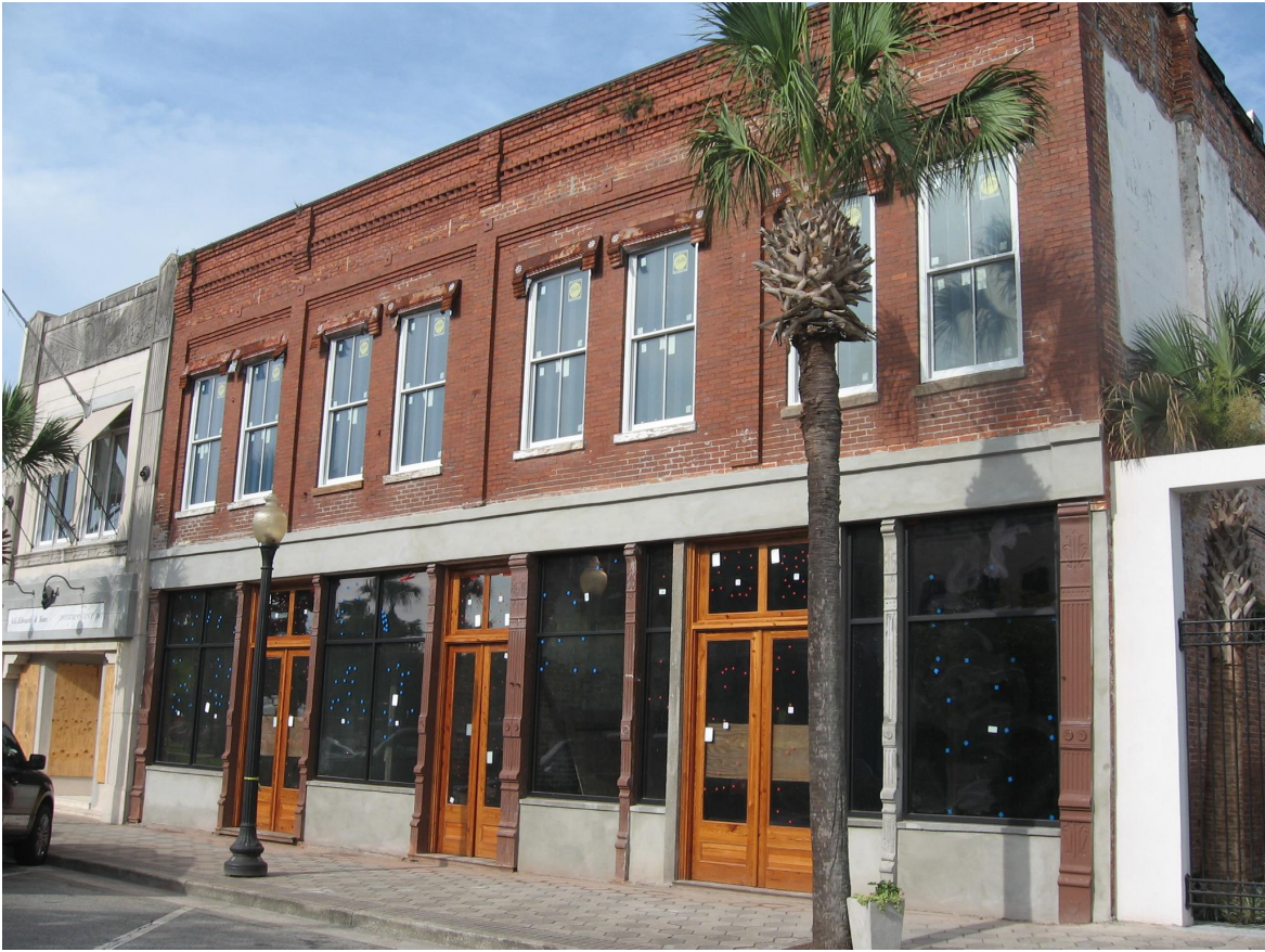
The rehabilitation of 1315-1317 Newcastle Street included the hardening of the bulkheads (the panels beneath the display windows) through the installation of brick and a concrete surface to withstand flooding.
