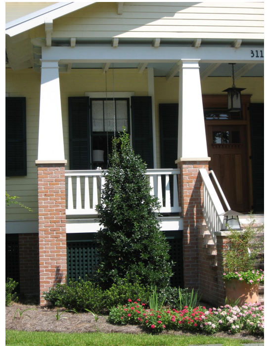
When elevating dwellings the porch columns may be extended on brick piers with lattice panels between the piers.
