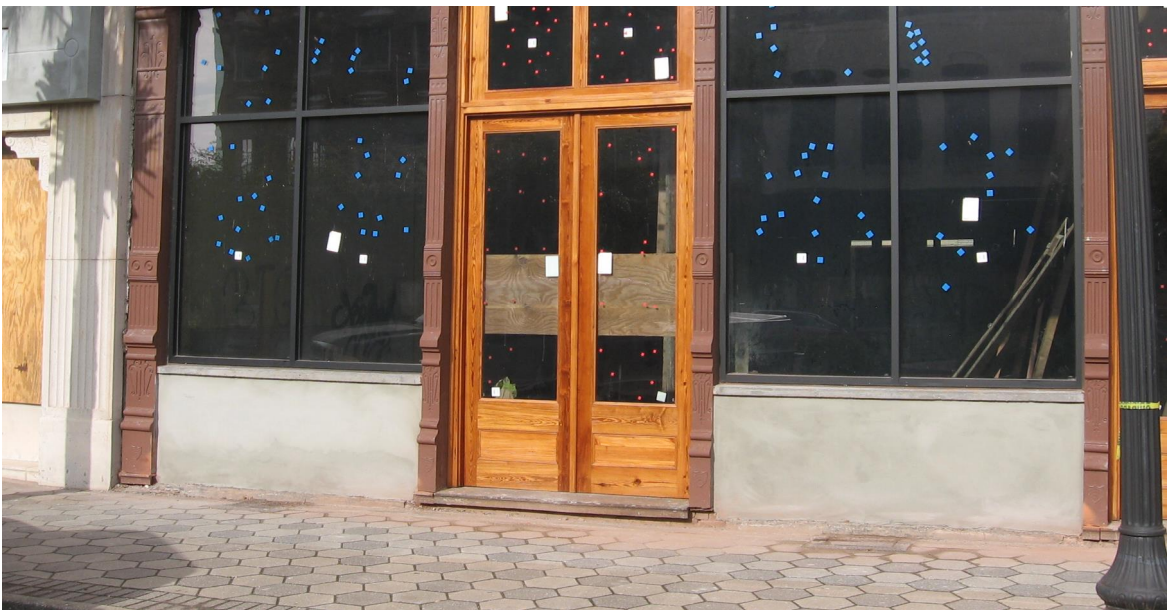
The rehabilitation of 1315-1317 Newcastle Street included the hardening of the bulkheads (the panels beneath the display windows) through the installation of brick and a concrete surface to withstand flooding.
