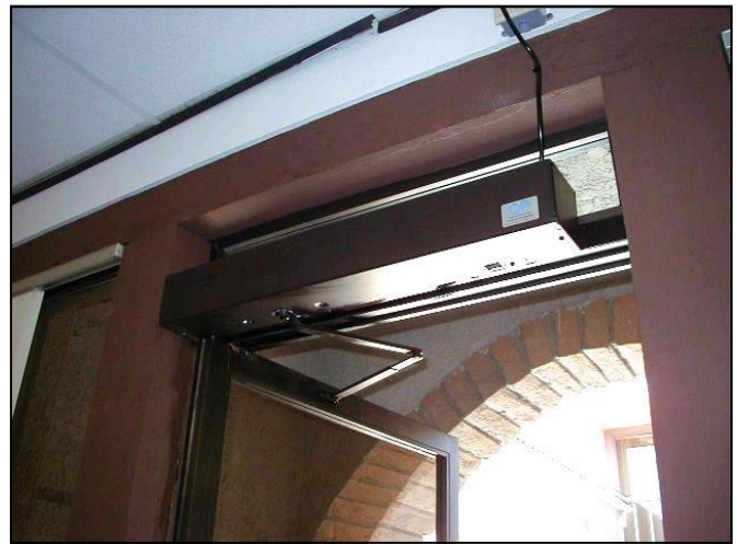
If needed, doors on commercial buildings can generally be retrofitted with push plates (left) which activate door openers (right) to allow wheelchair access.
