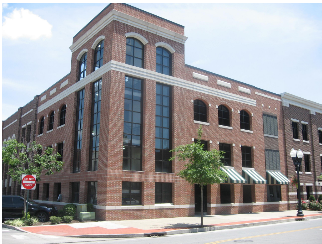
Any proposed parking garages should also be designed to be compatible with the historic character of the commercial district. This example has traditional window and door openings, awnings and cornices at the roofline.
