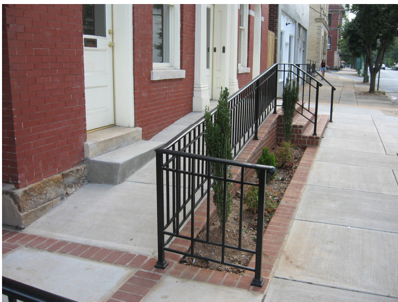
If a grade change is needed for access, construction of a concrete and metal ramp screened by landscaping may be an acceptable alternative (left). When non-historic storefronts are remodeled, new traditional storefronts should be designed with lever door handles and appropriate widths (right).
