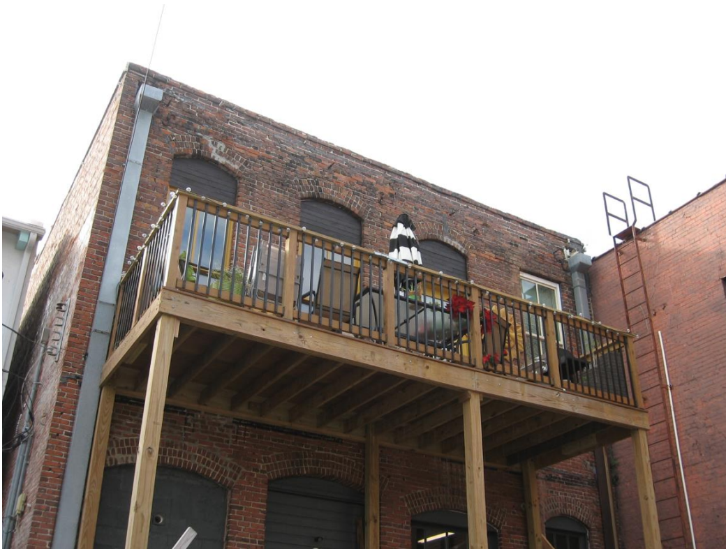
This rear deck is of appropriate design of wood construction and with simple balusters and railing (1604 Newcastle Street).
