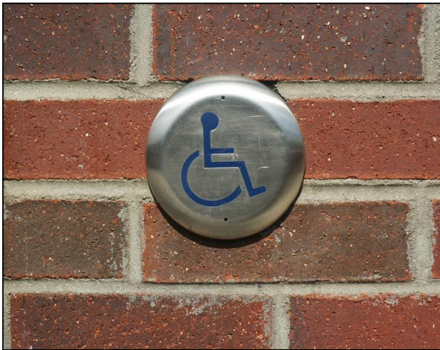
If needed, doors on commercial buildings can generally be retrofitted with push plates (left) which activate door openers (right) to allow wheelchair access.
