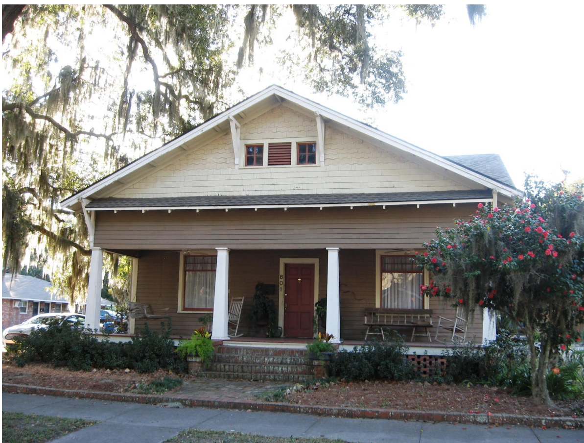
This Craftsman dwelling at 801 Albany Street has a deep, full-width porch with tapered posts, and eave brackets, character-defining features of this style.
