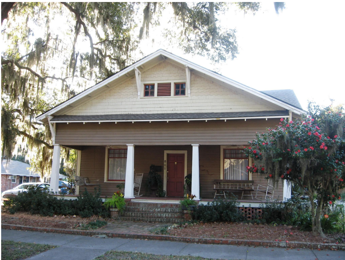
This Craftsman dwelling at 801 Albany Street has a deep, full-width porch with tapered posts, and eave brackets, character-defining features of this style.
