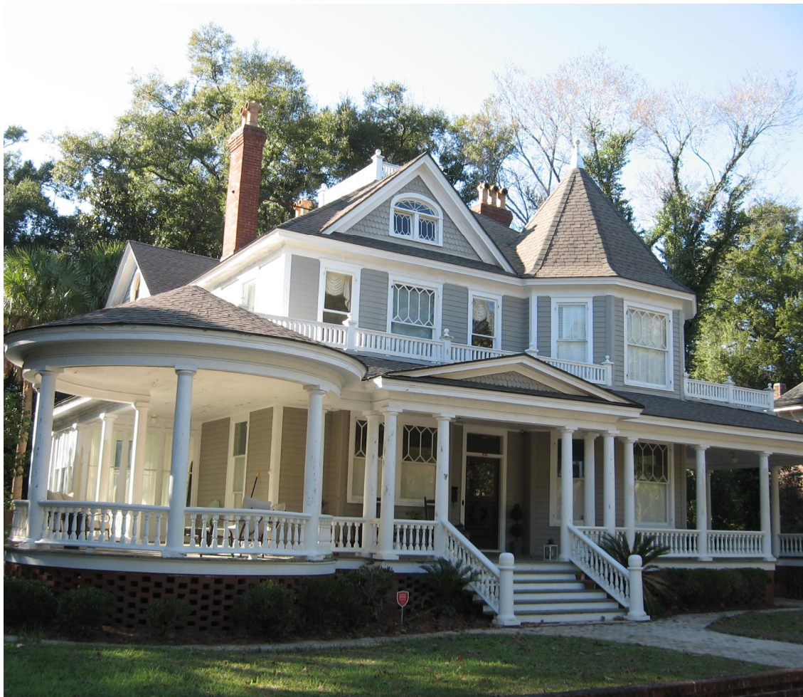
The Queen Anne style dwelling at 721 Union Street features a wrap-around porch and corner tower.
