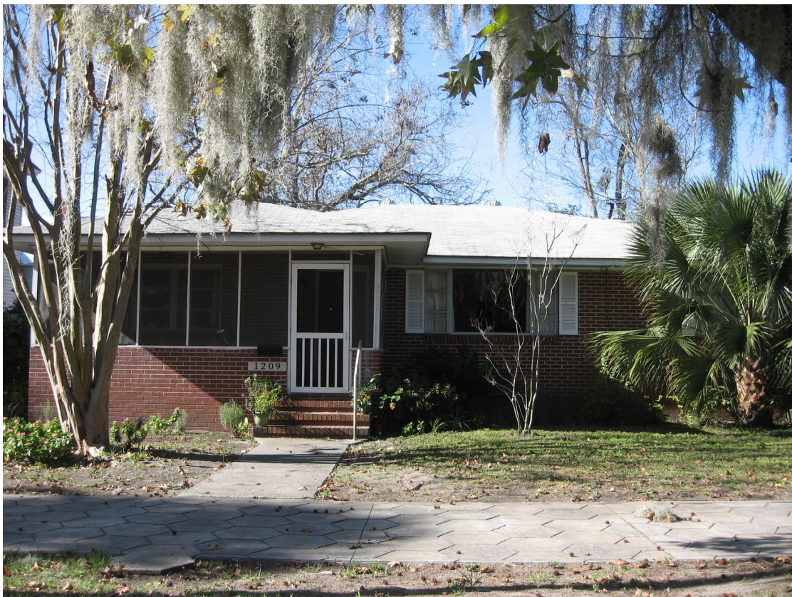
The Ranch plan dwelling at 1201 Union Street has a horizontal form, low-pitched hipped roof, and screened porch.
