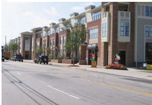
Figure 2.1 Mixed-use development helps to activate public streets
