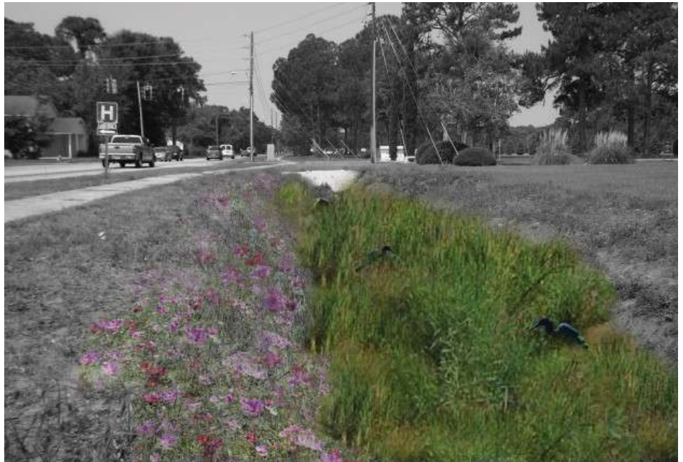
Improvements to the bioswale along Fourth Street
