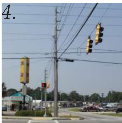
2. Streetscape, signage, and curb cuts along Altama Avenue 3. Altama Avenue center median near intersection with Community Road 4. Typical string mounted traffic signals
