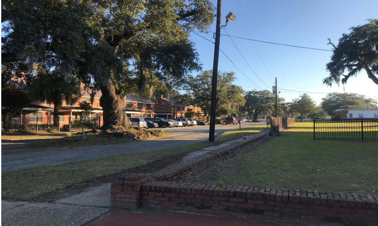
Picture 7 – ENE angle I Street (adjacent street)
