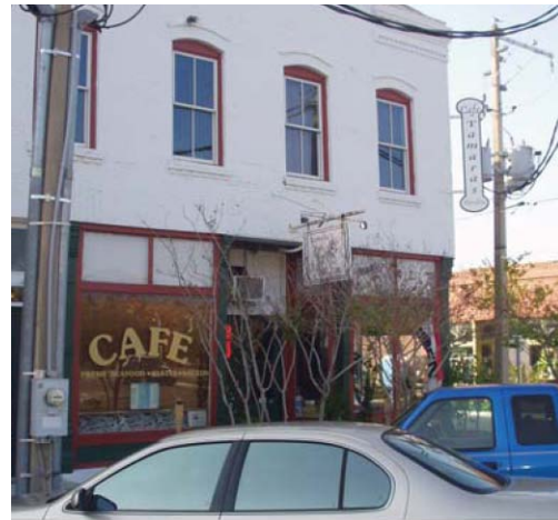
Figure 2.11 Corner stores contribute to a sense of place
