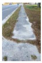
The photo to the left shows grass grown into the sidewalk joint that creates a potential fall hazard. The sidewalk should be weeded and edged. We do not provide this type of work since it is normally the responsibility of the property owner.
