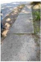
The photo to the left shows a displacement that is too big for our process. It is well over 2" high. Removing the high concrete will leave a slab that is too thin and susceptible to breaking. This sidewalk panel should be replaced with new concrete. Because we do not provide concrete construction services, this is not work we can provide. It will require your own concrete team or a general contractor.
