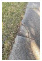
This next photo shows an example of a repair that is included in this repair offer. When we find a single broken corner such as this with a displacement 1" or smaller we will apply our repair process to create a flush joint at the cracked sidewalk.
