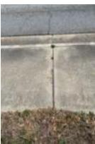
The photo to the left shows a joint that is chipped and can be filled. We do not fill gaps because most of our clients can do it less expensively with their own staff and materials purchased locally.
