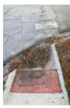
This next photo shows an ADA ramp that should be improved. There is a huge displacement of asphalt at the base of this ADA ramp that should be removed. It is not work we can provide.
