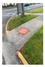
The photo to the left shows a loose truncated dome pad that should be replaced. This is not work we can provide.
