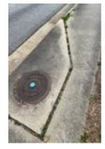
This next photo shows a wide gap between basin and sidewalk that should be filled. We do not fill gaps because most of our clients can do it less expensively with their own staff and materials purchased locally.
