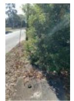
The photo to the left shows a basin lid with a displacement that is over 1" high. We cannot make a cut this large on a basin lid because of the rebar inside, and the position of the manhole does not allow us to cut an ADA compliant slope. The sidewalk around this basin should be replaced with new concrete. Because we do not provide concrete construction services, this is not work we can provide. It will require your own concrete team or a general contractor.
