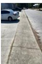
The photo to the left shows a stretch of sidewalk that is non-compliant due to a side-slope that is too steep. The length of sidewalk should be redesigned and replaced but it is not work with which we can help.
