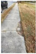
This next photo shows an example of broken sidewalk that should be replaced with new concrete. Because we do not provide concrete construction services, this is not work we can provide. It will require your own concrete team or a general contractor.
