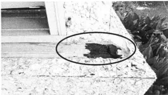
--- Wood rot on window and lower wall trim in several areas ---
