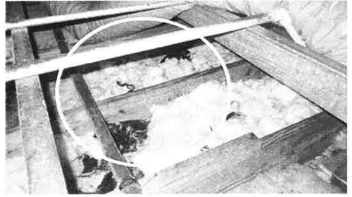
--- Attic insulation at front section missing; insulation over back area thin, approx. 2" ---
