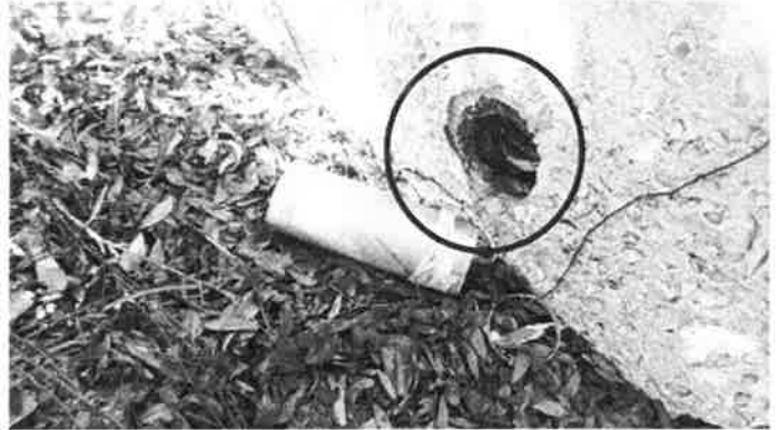
Dryer vent duct missing / removed, no cover
