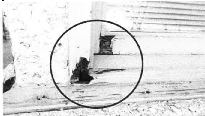
--- Wood rot on window and lower wall trim in several areas ---
