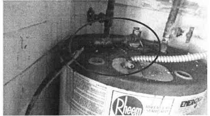
--- Water heater in garage utility at end of life – rusted and corroded, relief valve drain pipe too short ---
