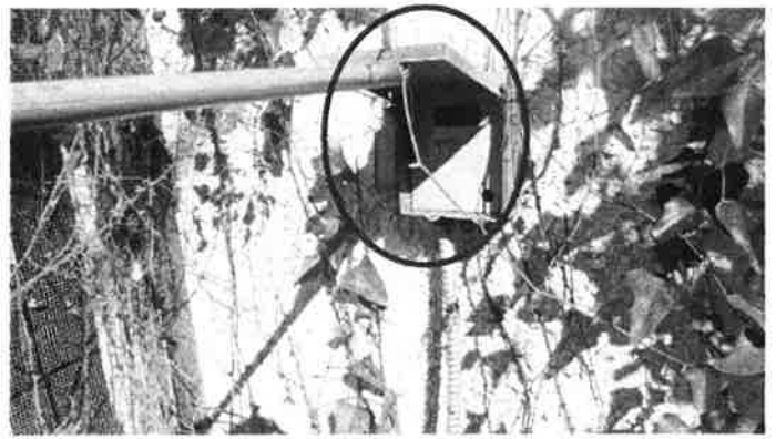
--- Both HVAC heat pumps / compressors removed / missing – electrical disconnects missing parts, damaged ---
