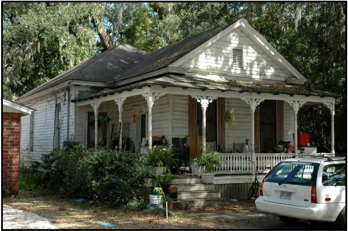
Photo 7: 722 Carpenter Street (c1895-04)
