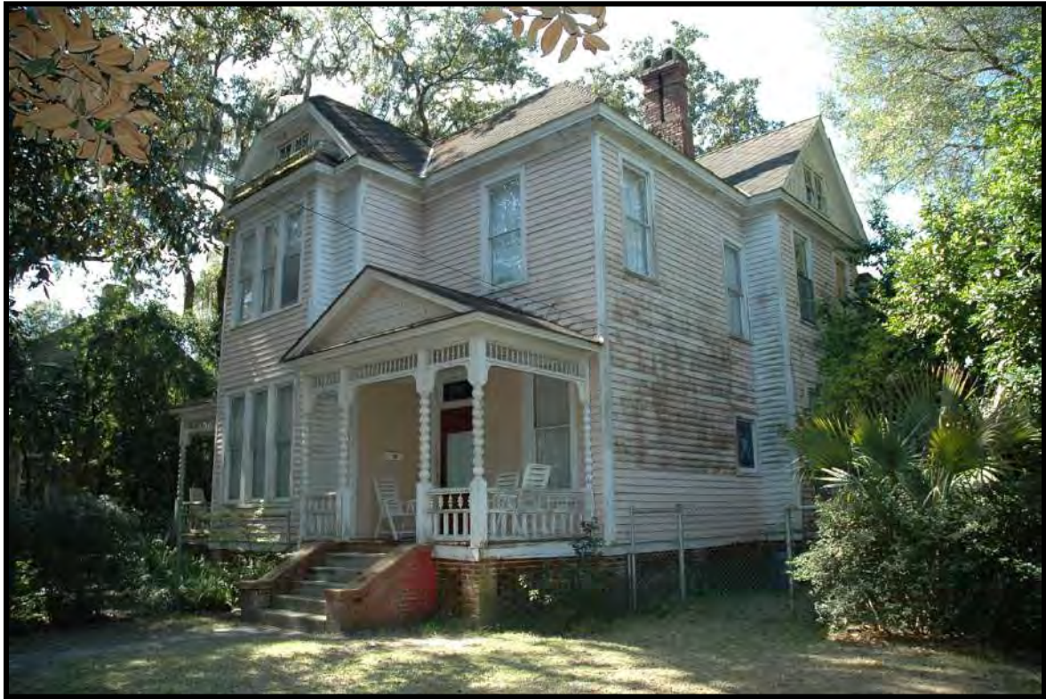
Photo 5: Spindlework Queen Anne Subtype - 915 Egmont Street (c1900)
