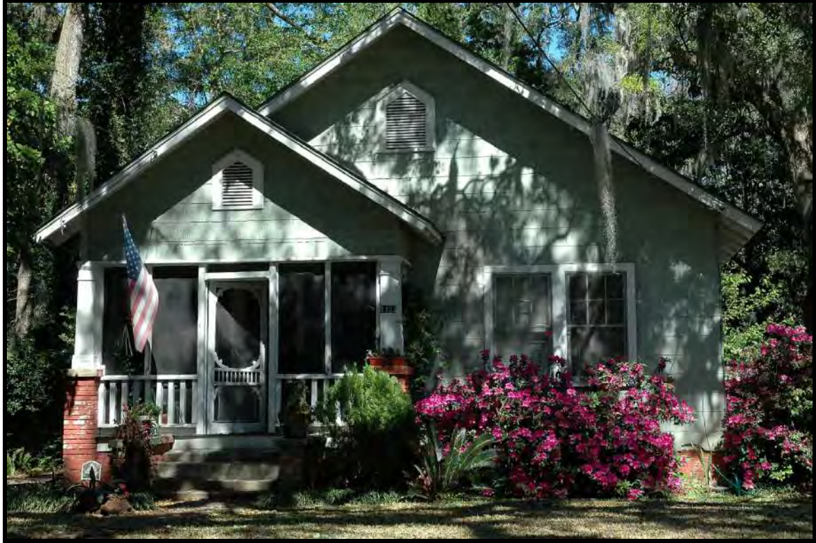
Photo 12: Front gable bungalow – 1303 Dartmouth Street (c1920-29)
