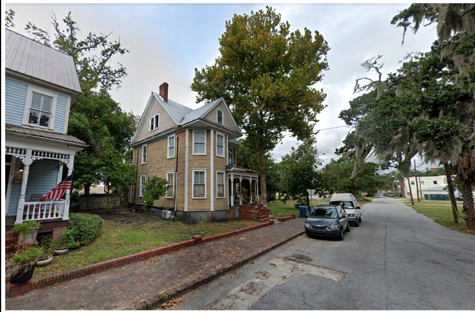
2 VIEW OF EXISTING BUILDINGS ON GRANT STREET PH1.1
