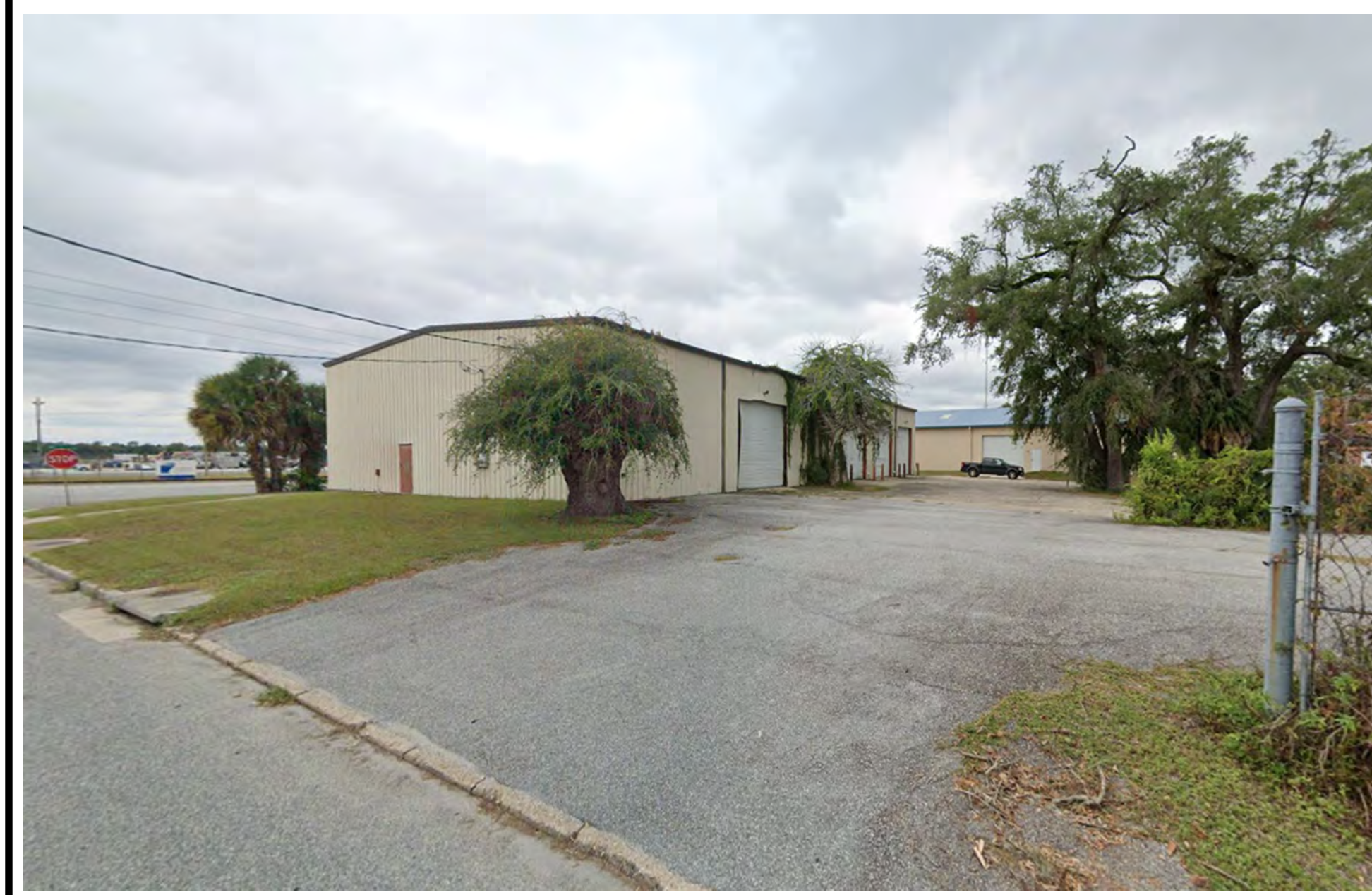
9 VIEW OF ADJACENT BUILDING ON HOWE STREET AND US-341 RH1.2
